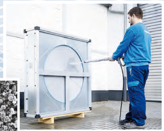
The storage mass with DekaTru® coating technology can clean with high pressure water cleaning.
