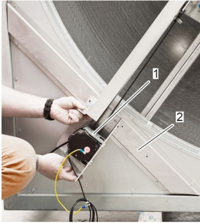
Fig. 34: Align the motor-side end of the cleaning rail
