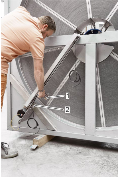
Fig. 38: Cleaning carriage bottom position
